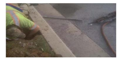
3) Lay the wire in the slot. Pour the epoxy over the wire and then compress Backer Rod (an easy to compress rope-like celled foam) over the epoxy. The probe end and the sealant should be no more than 1/4 inch to no less than 1/8 inch below the surface of the asphalt so that snow plows won't pick them up. Do not place backer rod over the tip, however, the tip should be sealed with a slight layer of epoxy.
